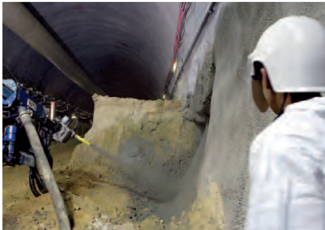
Application of sprayed concrete after excavation
