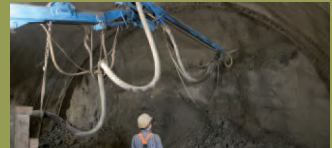
Remote controlled sprayed concrete application to stabilise upper bench
