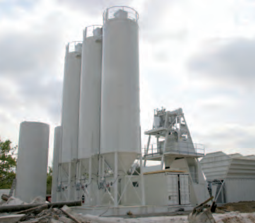
▲ Sellafield – nuclear construction
