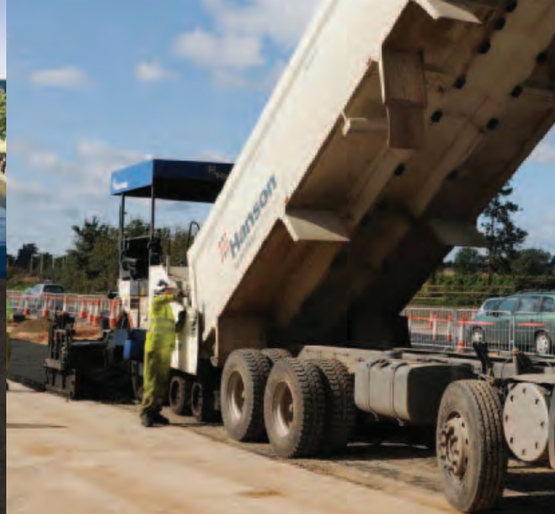
▲ A40 – infrastructure and road surfacing
